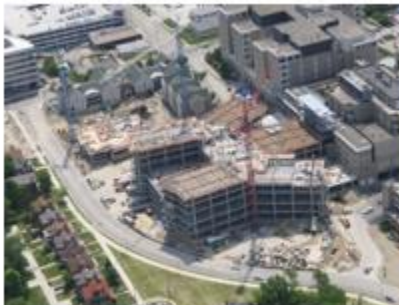
June 2019 Aerial View
