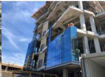
Glass Exterior Install
